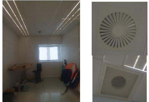
Figure 2 Window in test room (left) and ventilation original supply inlet (top right) and exhaust outlet (bottom right)
