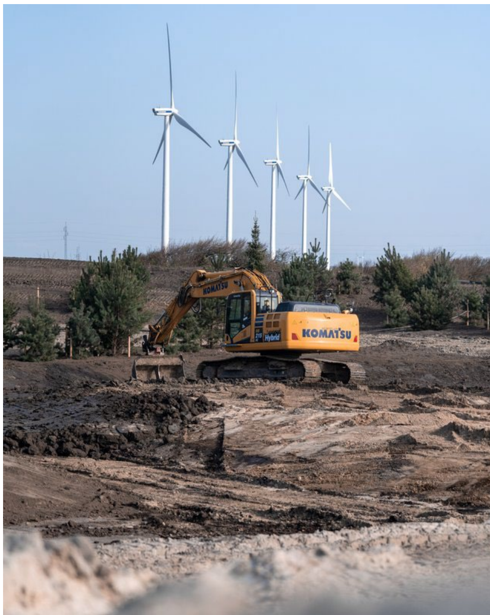
Illustration 1: Construction site, Naturkraft, 2019. Photo by Bjørn Ellermand, Naturkraft
