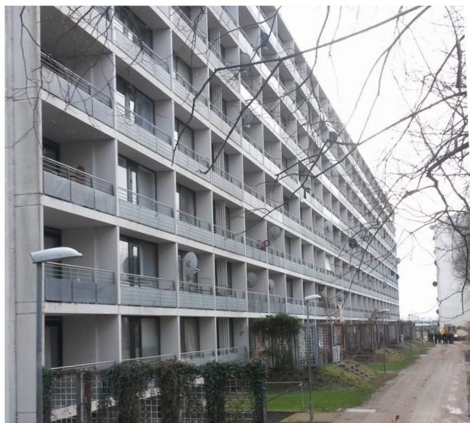
Figure 65 West facade - Gellerupparken.
