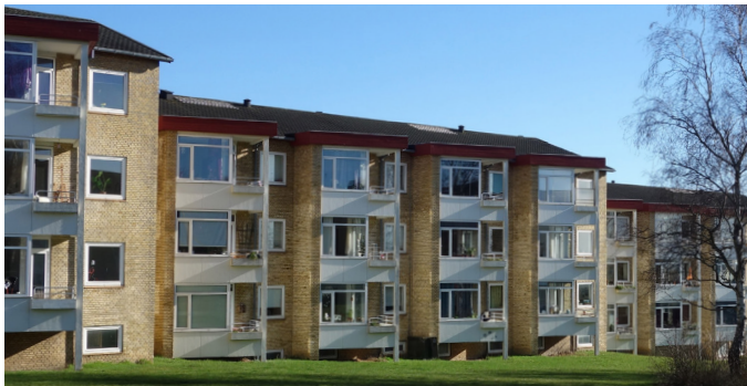
Figure 64 West facade - Søvangen.
