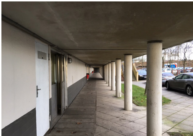
Figure 113 Existing threshold at ground floor level (East facade).
