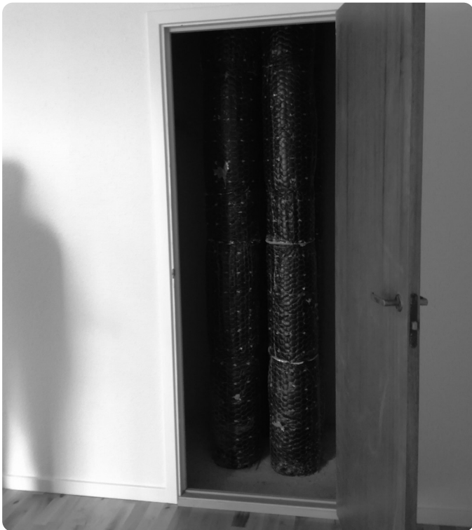
Figure 58 Ellebo. Two interior photos of ventilation pipes (left) and ventilation aggregate (right) in the same apartment. When implementing energy efficiency measures, we risk losing existing values (closet space) in efforts to add new ones (improved air quality).
