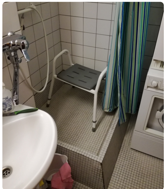
Figure 138 Existing bathroom in Toveshøj before renovation.
