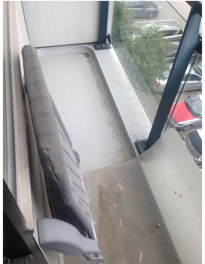
Figure 63 Single-room apartment with shallow balcony (Toveshøj).
