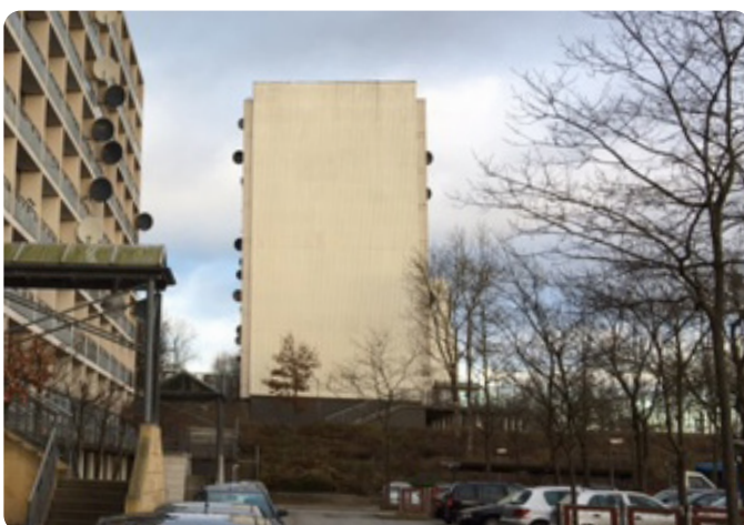
Figure 106 Gable facade before renovation.
