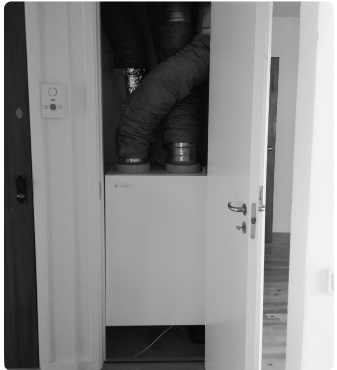
Figure 58 Ellebo. Two interior photos of ventilation pipes (left) and ventilation aggregate (right) in the same apartment. When implementing energy efficiency measures, we risk losing existing values (closet space) in efforts to add new ones (improved air quality).
