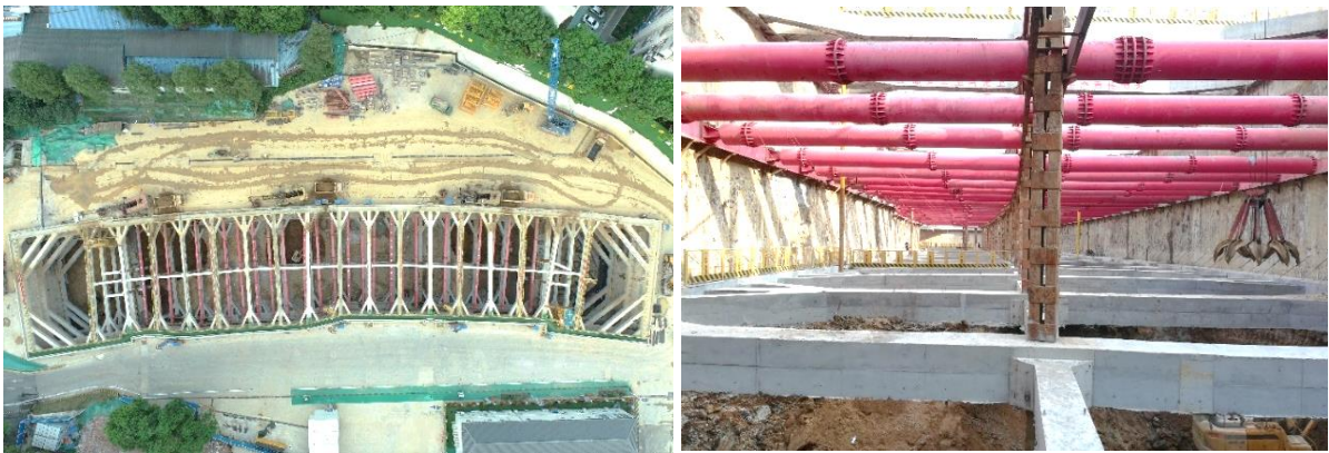
Figure 2: The Selected Deep Foundation Pit for Case Study.
