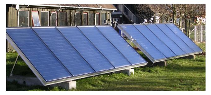
Figure 2 Flat-plate solar collectors used in Danish solar heating plants
