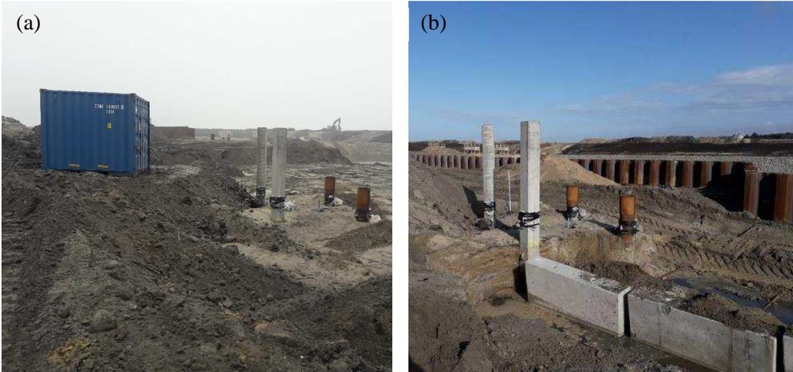
Figure 6. Test site at (a) Day 78 and (b) Day 126 (before placing the 3.0 m fill). The concrete slabs in (b) are anchor plates for the sheet pile wall seen in the background.
