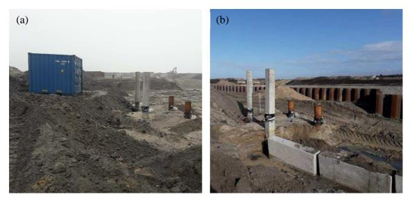
Figure 6. Test site at (a) Day 78 and (b) Day 126 (before placing the 3.0 m fill). The concrete slabs in (b) are anchor plates for the sheet pile wall seen in the background.
