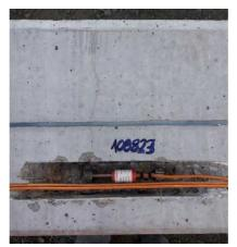
Figure 7. Installation of a DFOS cable and a VW on a precast concrete pile
