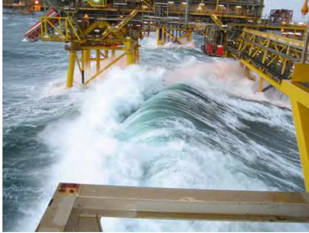
Figure 2.1: Plunging breaking wave at Tyra West, November 2017. Photo courtesy of Mærsk Oil.
