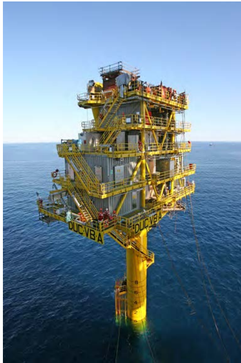
Figure 1.2: Target structure type. Photo shows the Valdemar BA 2006 well-head platform in the North Sea. Photo courtesy of Mærsk Oil.
