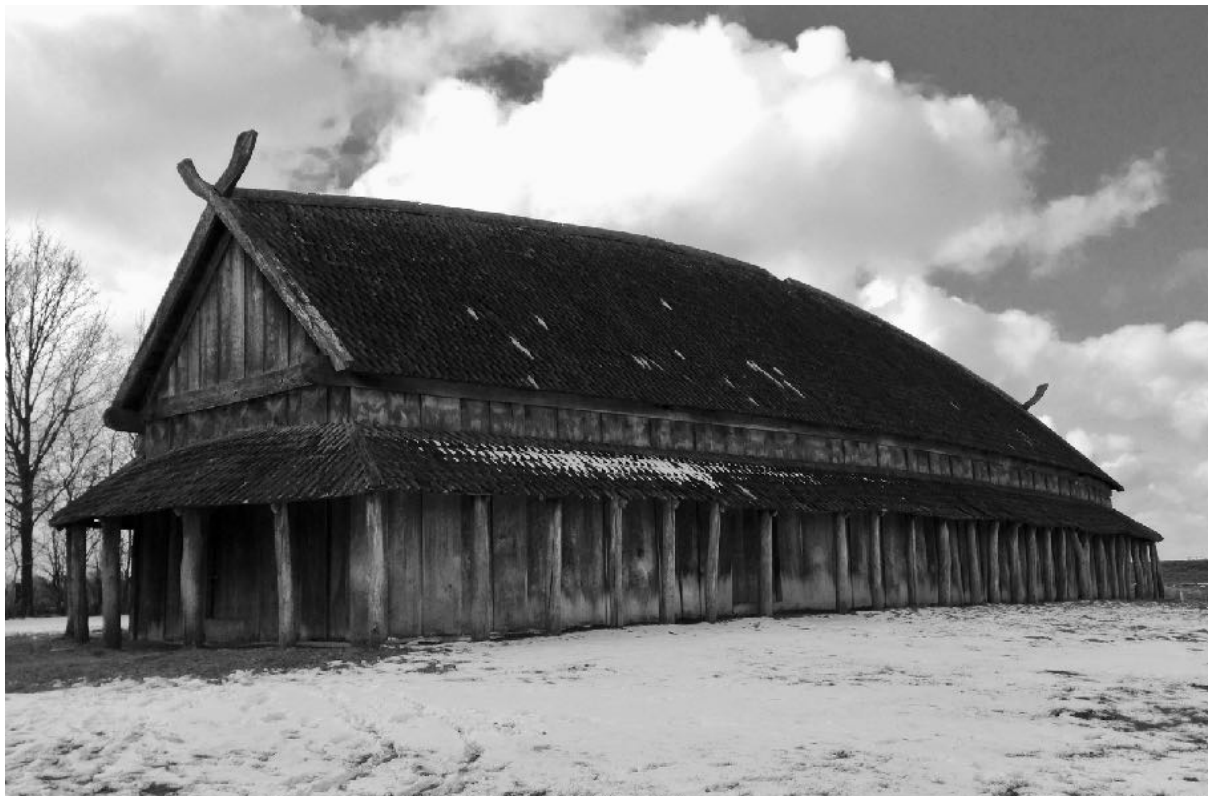
Figure 4: The earliest reconstruction of the Trelleborg house built in 1942 by architect C. Schultz, who also participated in the excavations at Trelleborg. The buttresses were interpreted as a gallery surrounding the building. Later excavations showed that the buttresses had been slanting towards the house and probably were a more integrated part of the house construction (photo by author).
