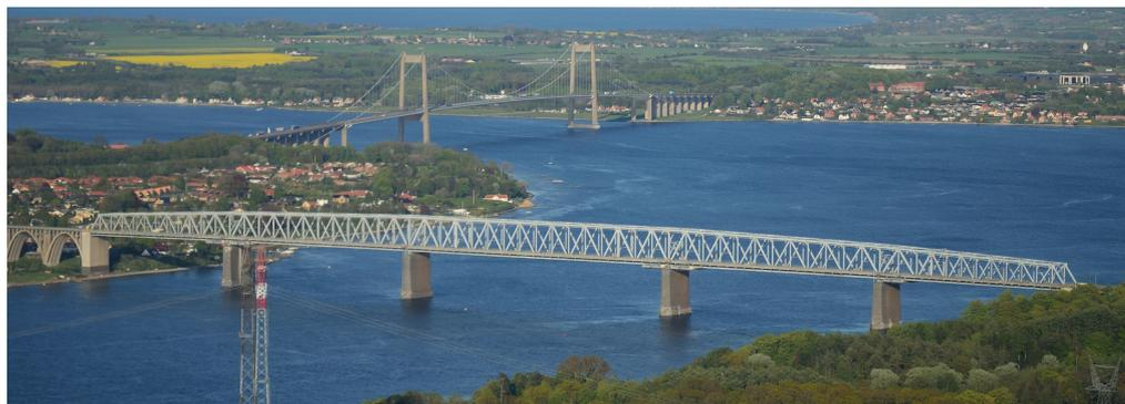
*Figure 9.5: Photo of the Little Belt Bridge from 1935. The settlements of the piers have been monitored closely since construction. Photo after (Colourbox 2017).*
