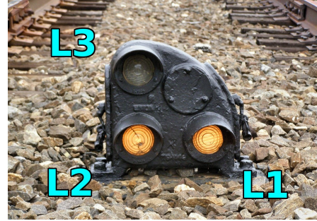
Fig. 5: Picture of railway signal, with lamps indicated
